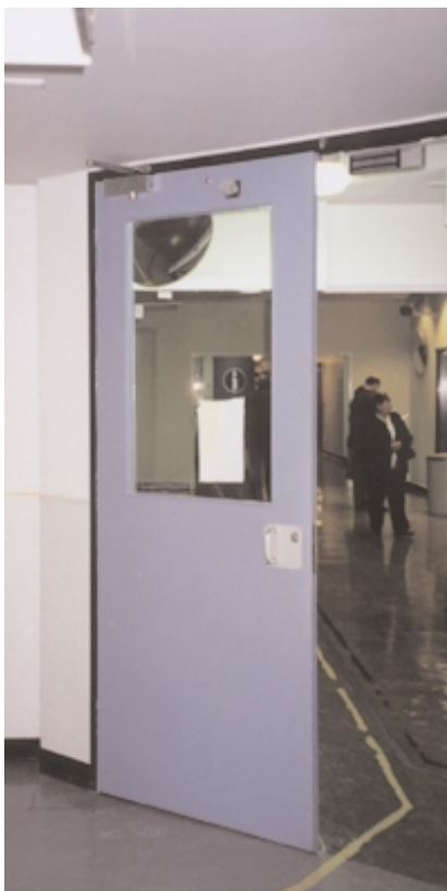
Evacuation is a primary concern during an audit.
